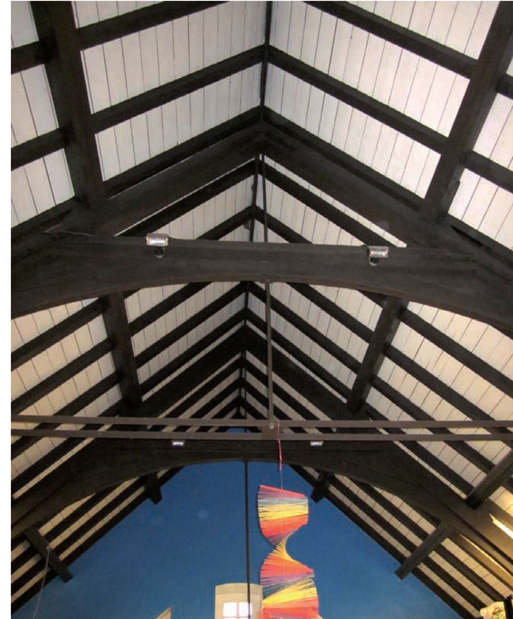
Clondalkin Library Roof
