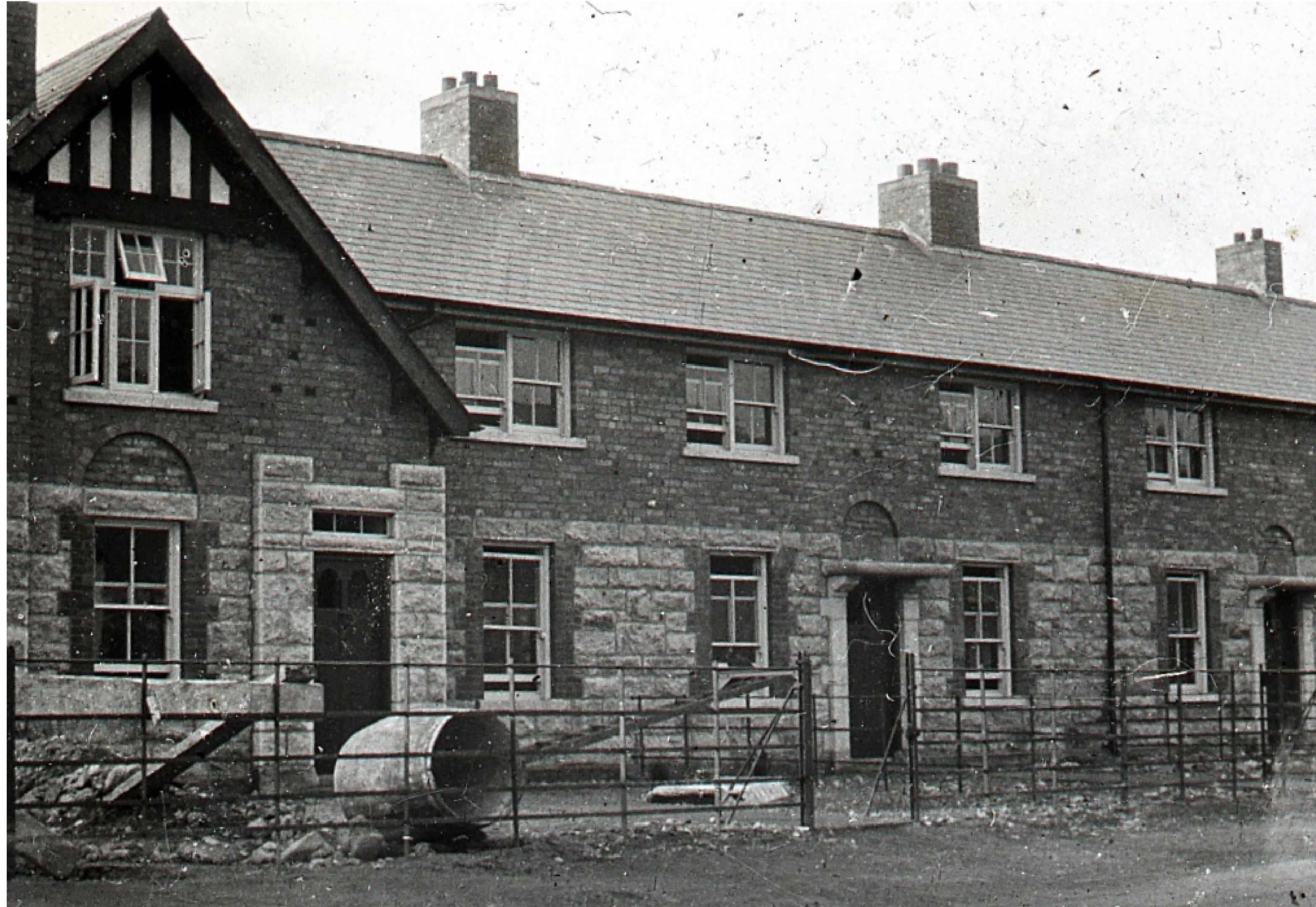
Chapelizod Housing in 1916
