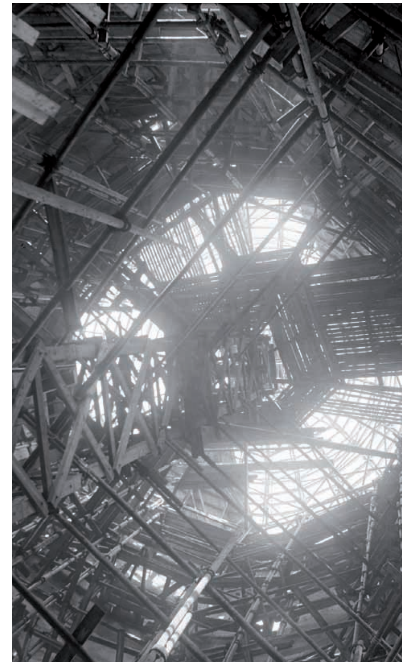
Four Courts scaffolding c 1926
