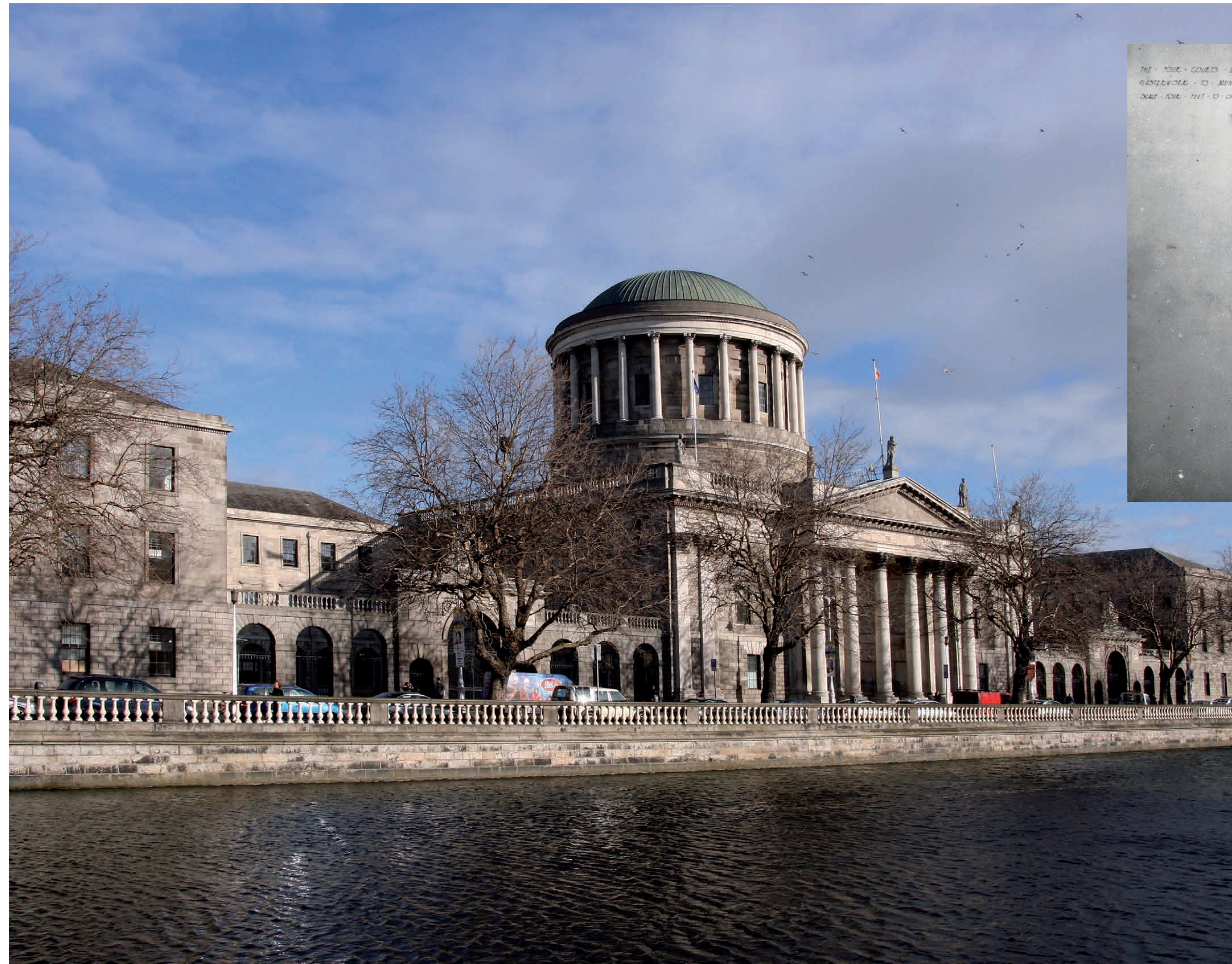
The Four Courts today
