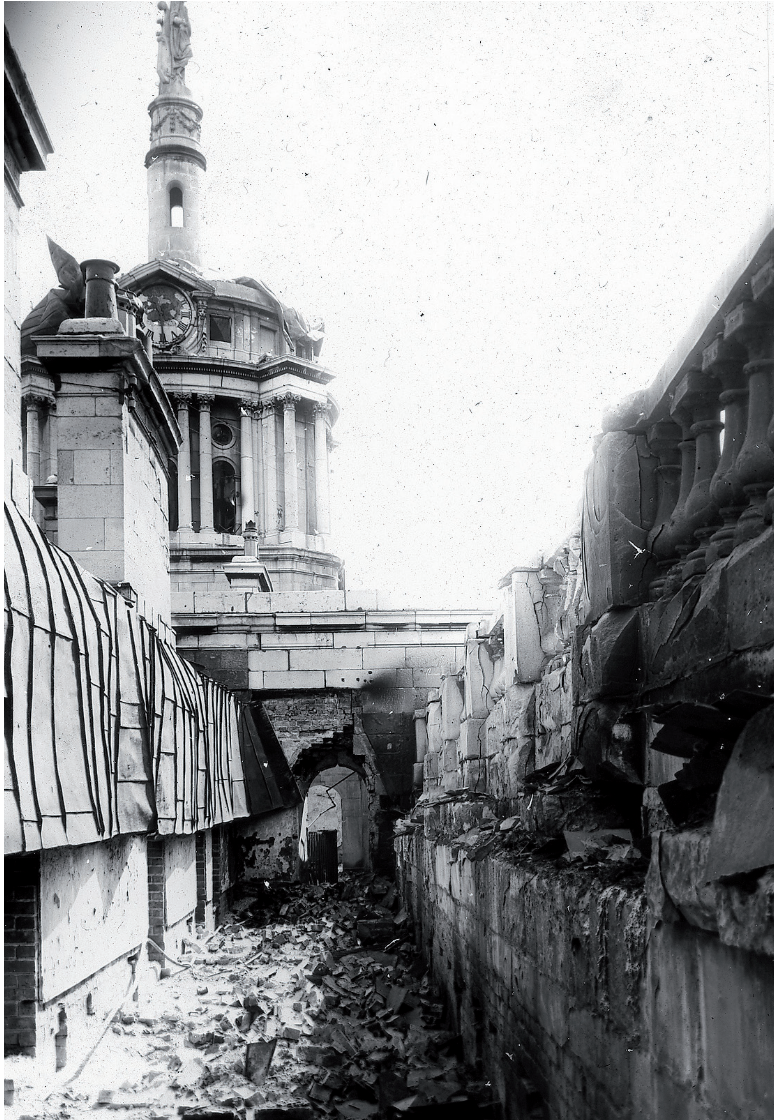
Custom House after fire May 1920
