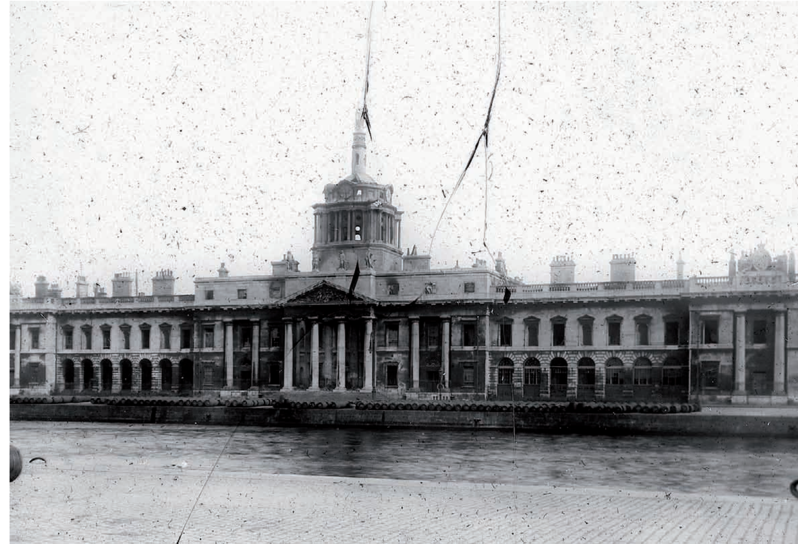
Custom House after fire May 1920
